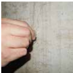
Hairline Cracks
